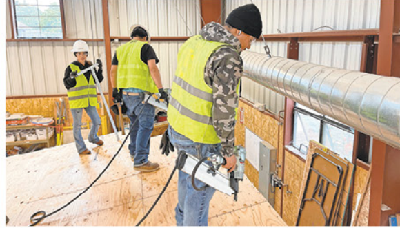
Three Rancho Cielo construction students at work on the Nexus 01 competition home.
